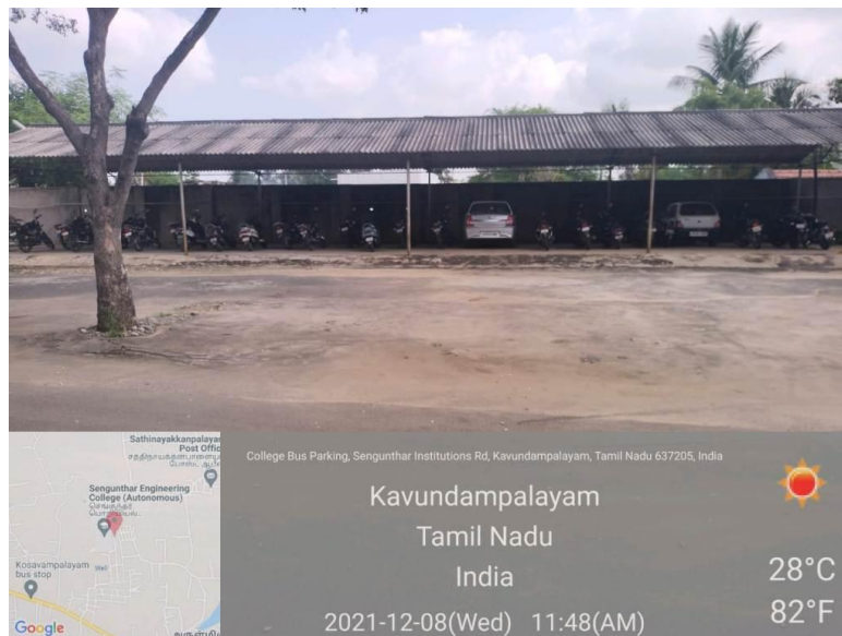
Vehicle Parking Shed for Two Wheelers and Four Wheelers
