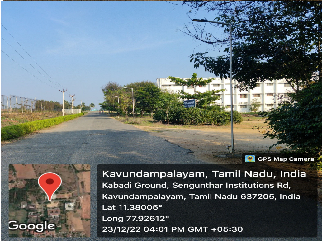
LED street lights in the campus roads
